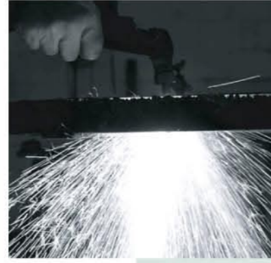
Fabrication shop, plasma cutting
